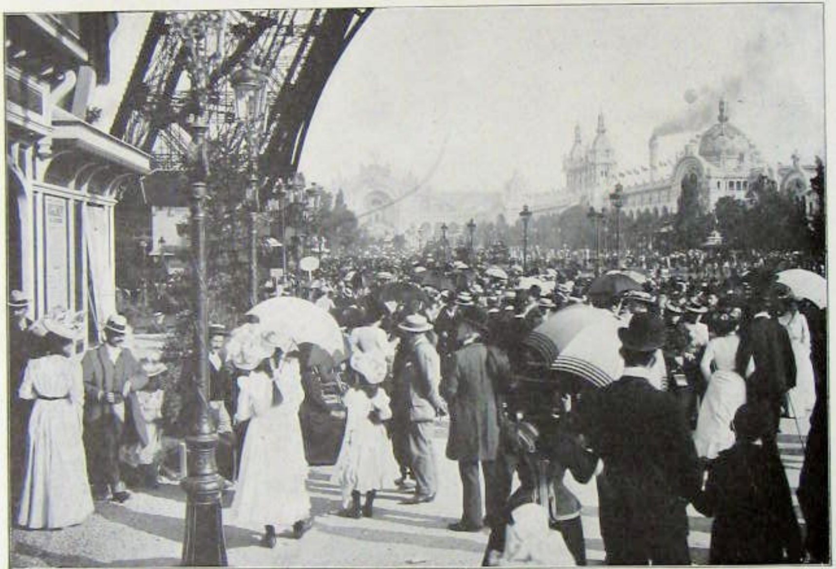
UNDER THE TOWER
