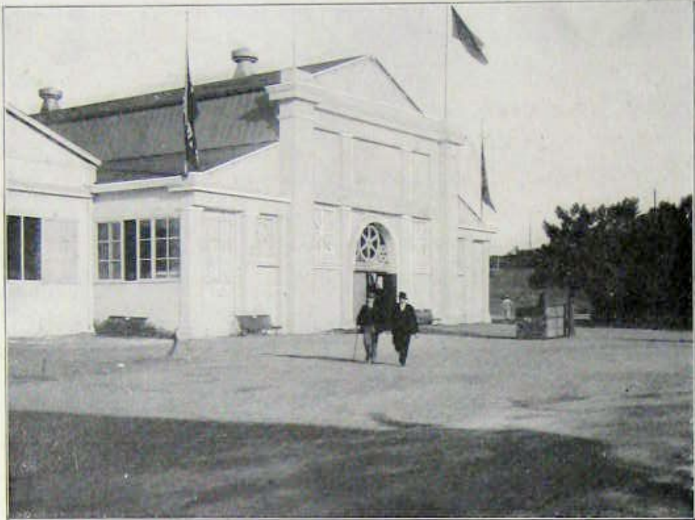
THE AMERICAN MACHINERY BUILDING
