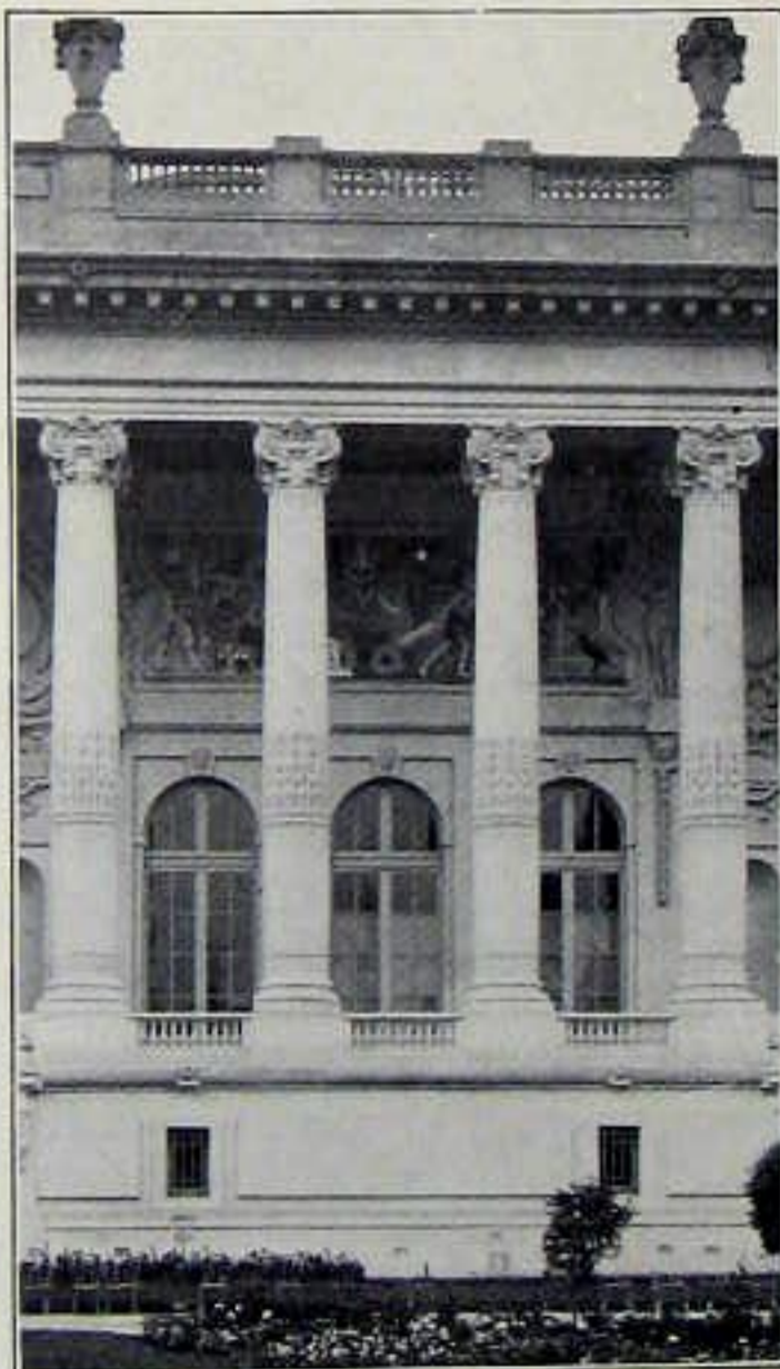
A FRAGMENT OF THE FACADE
