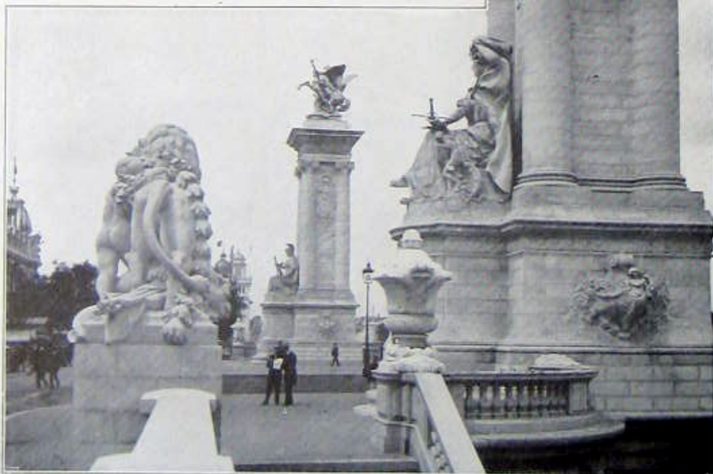
PYLONS OF THE BRIDGE
